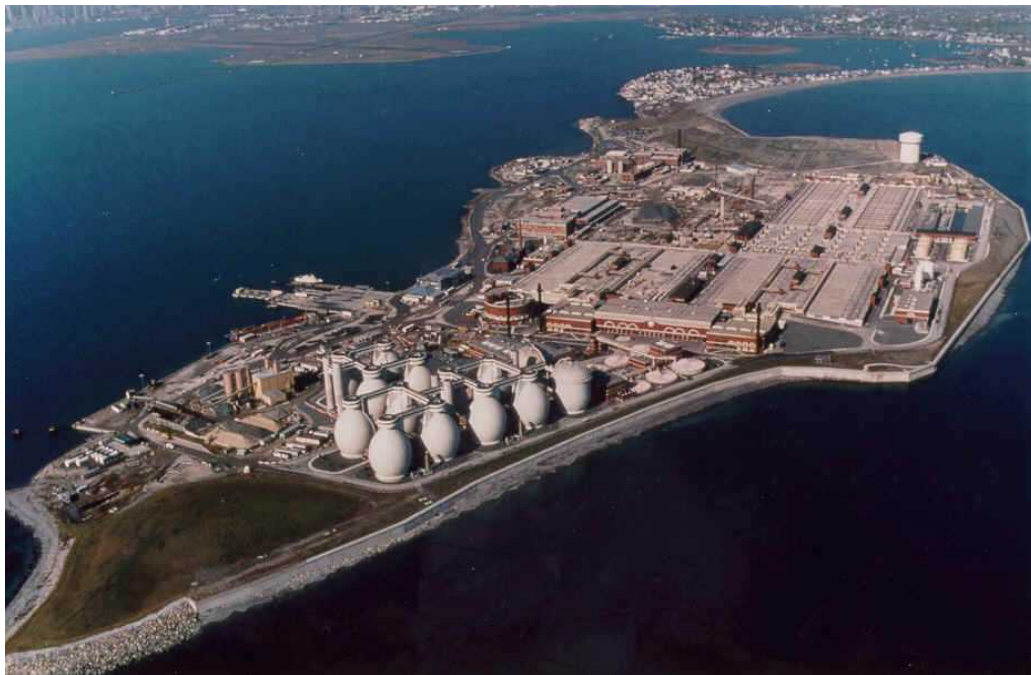
Aerial Photo - Deer Island Treatment Plant
